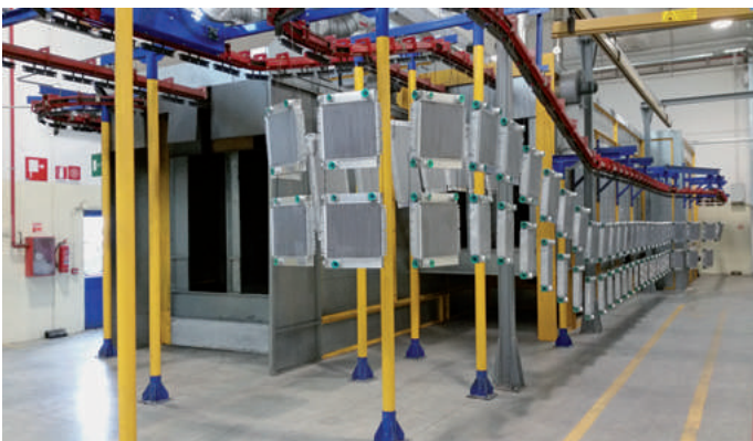
Paint shop (powder coating)
